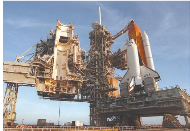
The Rotating Service Structure (left) is rolled open for launch. Entry to the Payload Changeout Room is exposed.
